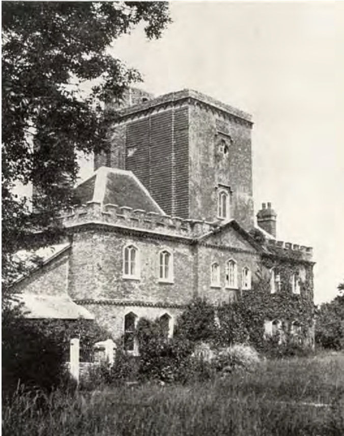
Laughton Place Tower, before wings demolished c.1925
